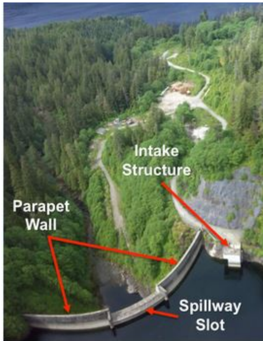
Dam 174' high x 430' wide Spillway 15' high x 100' wide
