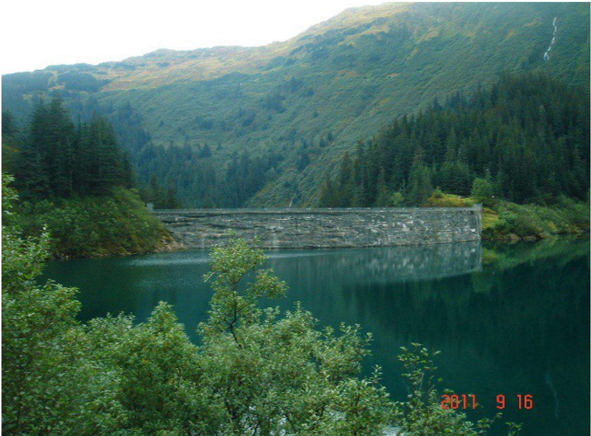
Upper (old) Power House
